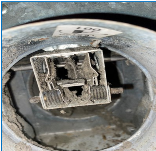
Fig No. 27— Damaged or twisted spring will prevent correct operation
