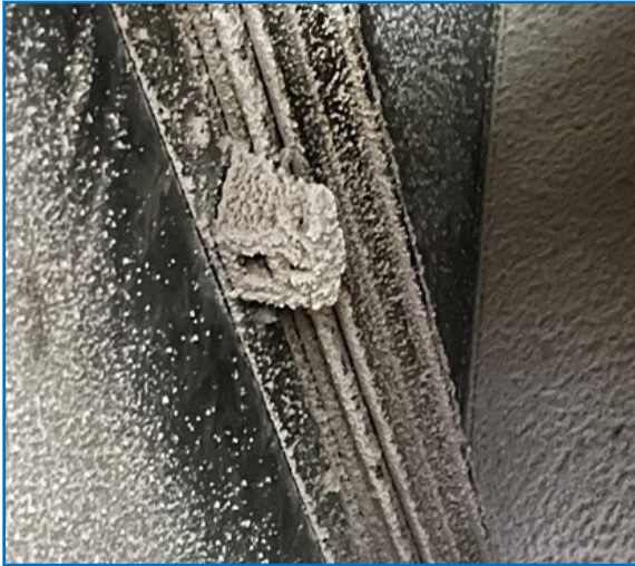
Fig No. 25— Fusible element will not operate at correct temperature due to insulating effect of debris
