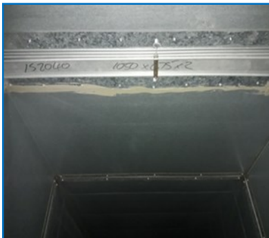
Fig No. 13— Hook and Fusible Bar
