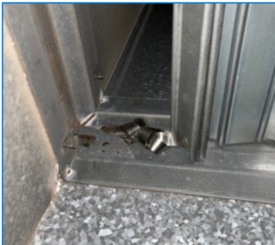
Fig No. 27— Damaged or twisted spring will prevent correct operation
