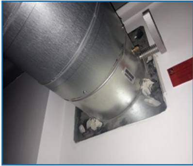
Fig No. 15— Single Blade/Spring Lever
