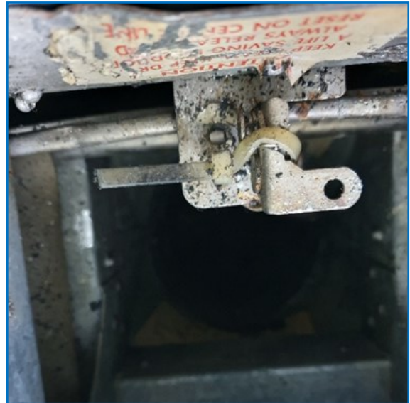
Fig No. 14 — Not to manufacturers specification must be a proper link
