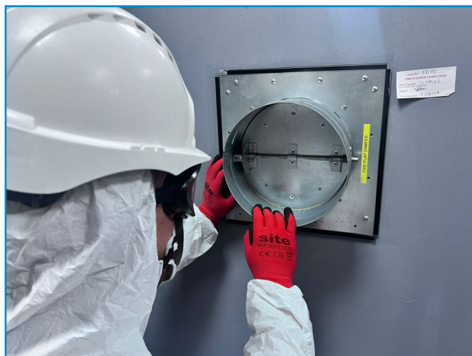
Fig No. 3,4,5 (L-R) — Functional Test
